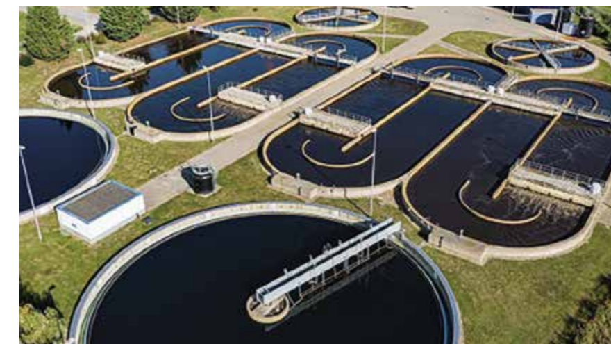
The MFC technology is being used on wastewater from wastewater treatment plants.
